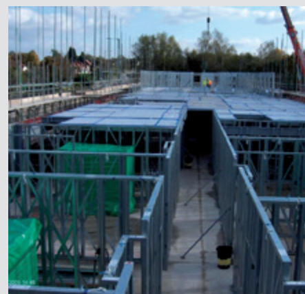
Wall panels installed with perimeter scaffolding
