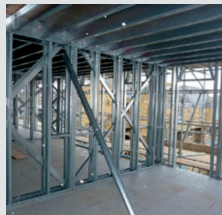
Wall panel supported by temporary struts
