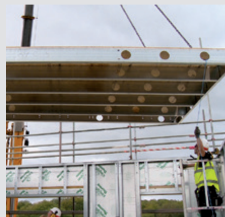
Installation of a light steel floor cassette
